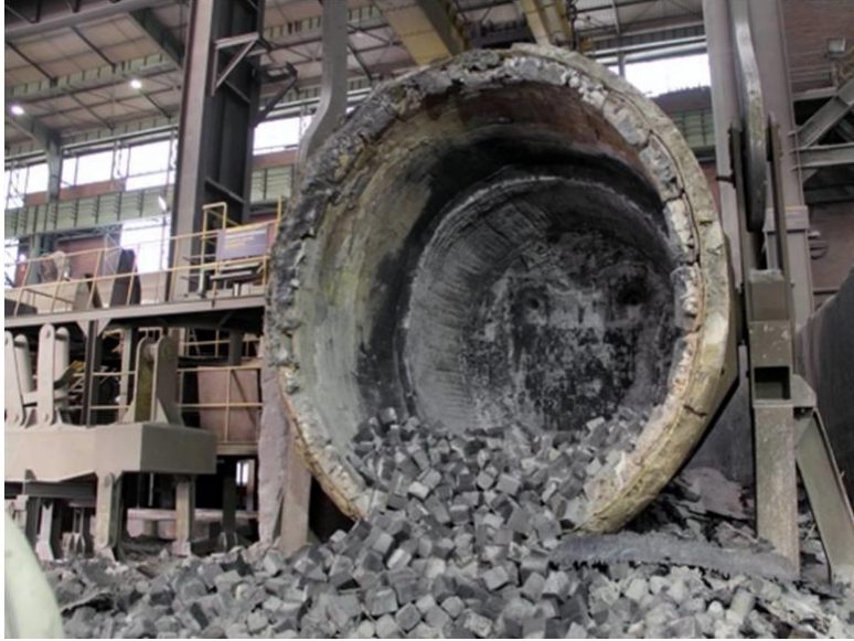
Fig 1: Periodically oven reconditioning exchanging high quality magnesite refractories (Sidenor Basauri)
